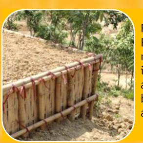
For many households in Potibunia mudslide is a major threat. CARE has identified the vulnerable areas and is constructing barrier walls to mitigate against erosion and slides.
