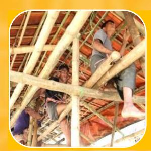
To help keep people dry and structures standing, CARE has disbursed shelter upgradation kits to 22,000+ people that contained bamboo, tarps, and rope etc. to strengthen the shelters from wind and rain.
