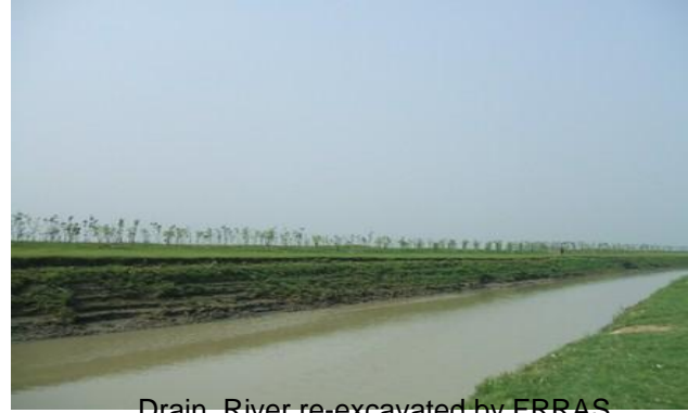
Drain, River re-excavated by FRRAS
