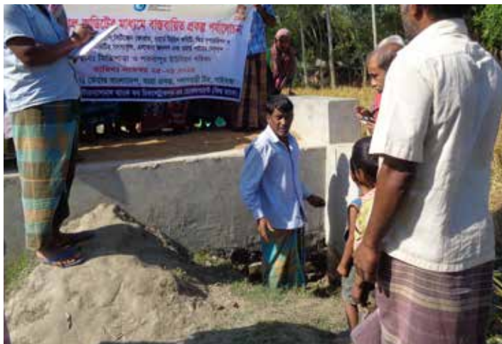
The box culvert before social audit
